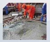
2 Assemble the reinforcement and install it in the formwork
